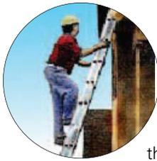
Non-self-supporting ladders, which must lean against a wall or other support, are to be positioned at such an angle that the horizontal dis-
