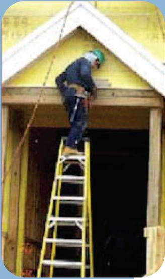
The height of the ladder is inadequate for this worker's job. Never stand on the first or second step of the ladder.
