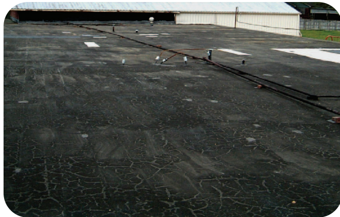
The roofing surface loses its elasticity and begins to look like cracked leather.
